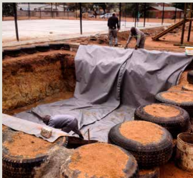
The community gardens in the Bontleng park pictured above are watered using the run-off rain collected in underground cisterns next to the futsal court. The photo below shows how the cisterns were constructed.
